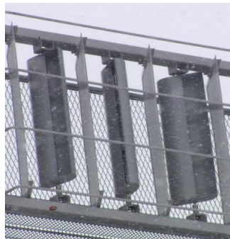
Fig.2 Small wind turbines suppressing visibility hindrance caused by drifting snow
