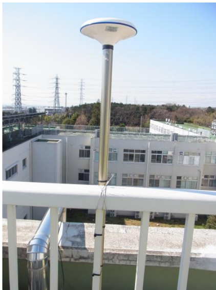
Fig.1 Base station antenna installed on the roof of a building in Numazu College of Technology.
