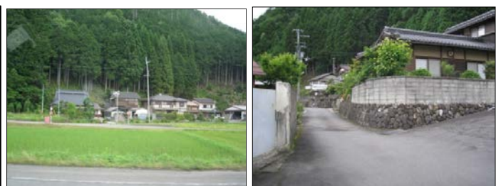
Fig.2 The potentially dangerous Housing (Place at Kyoto City)
