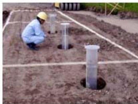
Figure-2 Measurement on embankment
