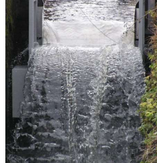
Fig.3 Micro hydraulic turbine installed at drop & power system interconnection equipment
